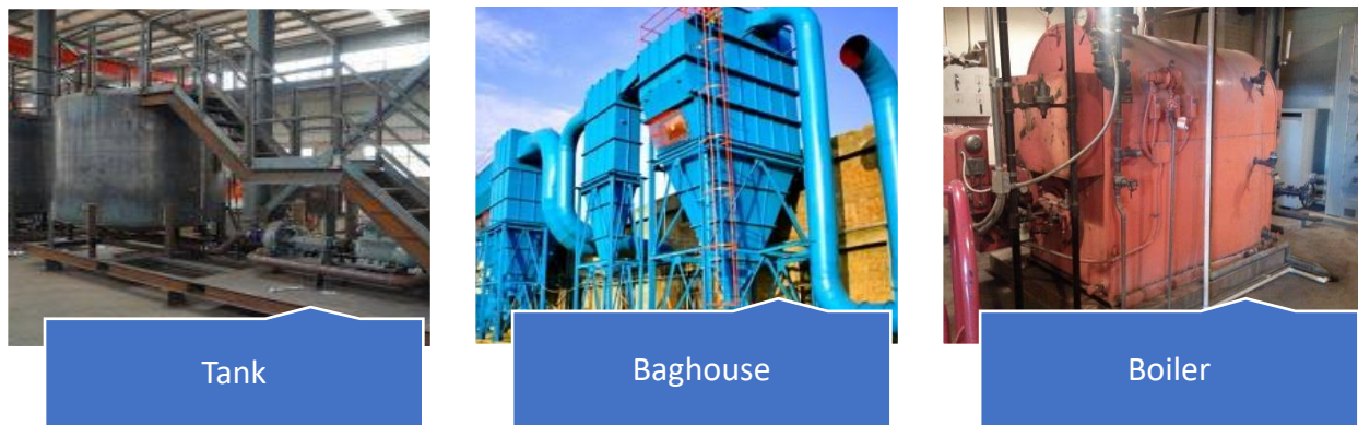
Figure 4-7: Examples of General Industrial Facility Equipment
