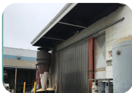
Cross-Draft Minimization Using Overlapping Strip Curtains
