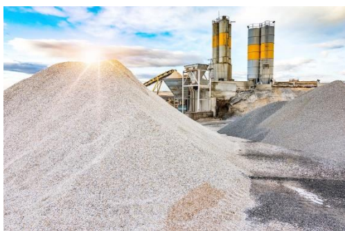
Figure 5f- 3: Aggregate or rock plant
