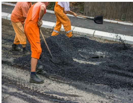
Figure 5-2: Asphalt being used for paving
