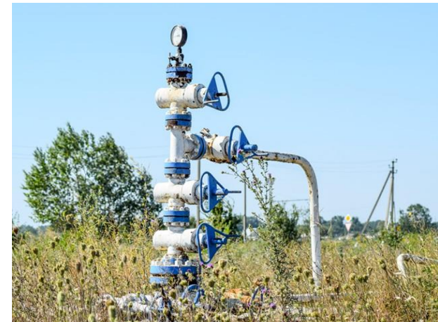
Example of an Injection Well
