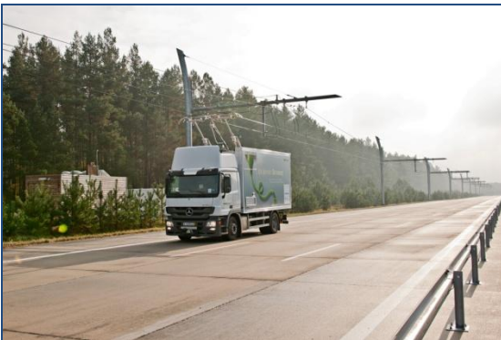
Figure 5 Truck Catenary (Siemens)
