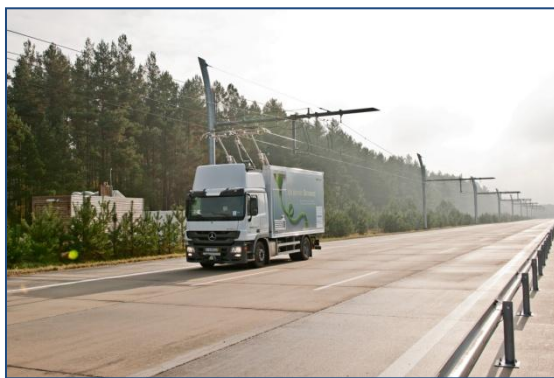
Figure 5 Truck Catenary (Siemens)
