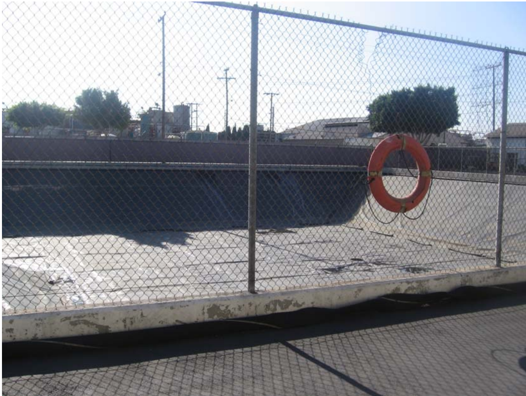
Figure 3-1 Storm Water Retention Pond Not In Use
