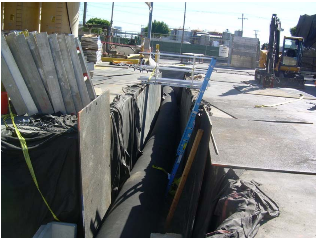
Figure 3-2 Current Replacement of Storm Water Piping
