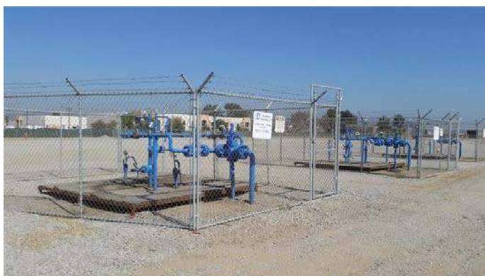
Figure 1-15. Typical Water Injection Well Located at 700 Block. For full size, see Figures section at the end of the Chapter 1.
