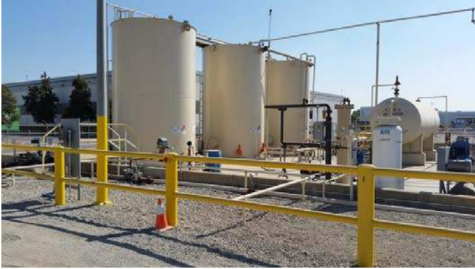
Figure 1-8. Existing Truck Loading Connection.
