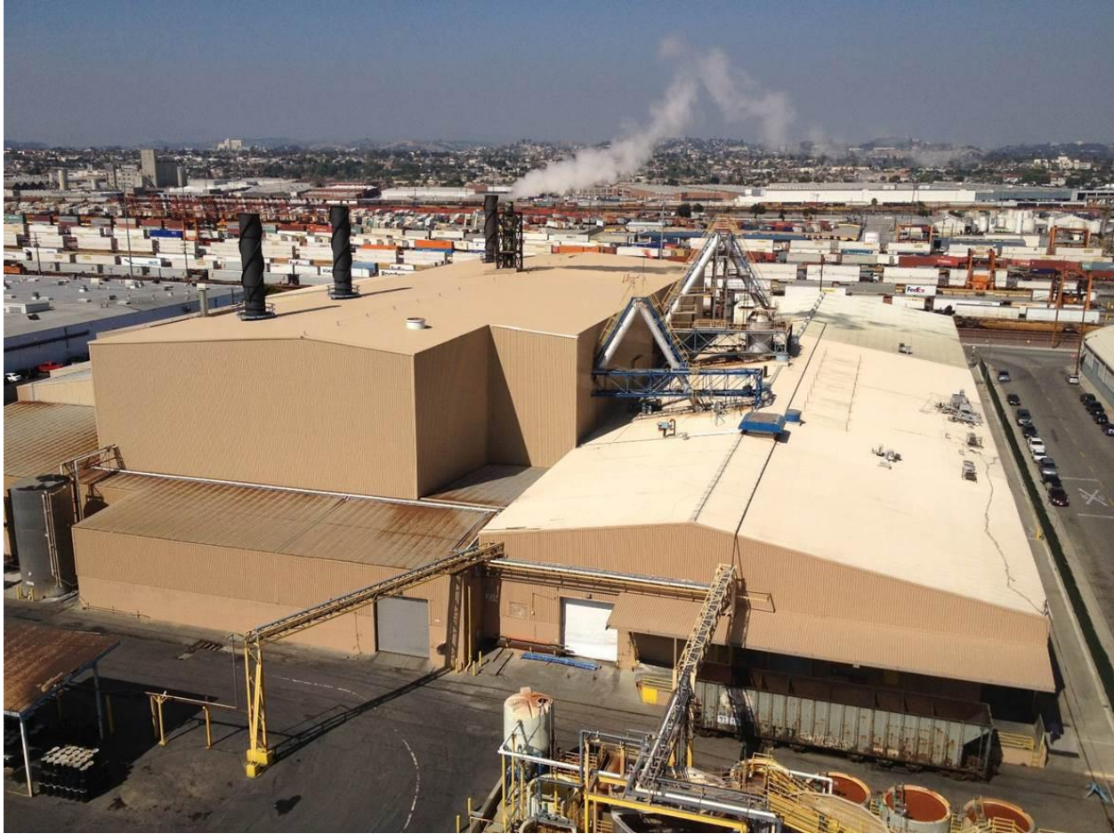
Figure 2-1 View of the Existing Exide Facility
