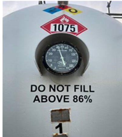
Figure 1. Photo of Tank #1 depicting maximum propane liquid fill volume
