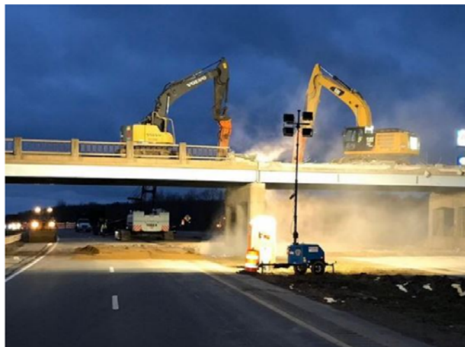
Figure 1-4 Bridge Demolition Activity Over a Large Roadway
