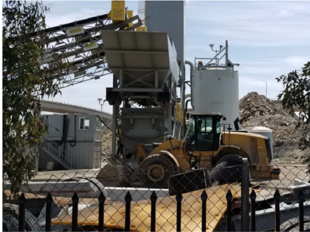
Figure 1-3 Portable Crusher at Roadway Project Near a Receptor
