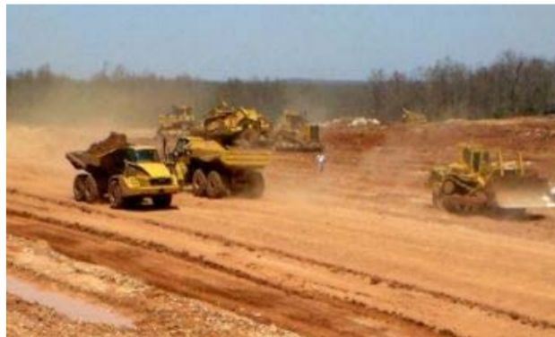
Figure 1-5 Earth-Moving Activities and Associated Fugitive Dust
