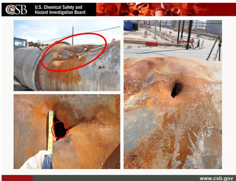
Figure 4 — Rupture of tank resulting from February 18, 2015 explosion at the Torrance refinery. The rupture shown in the lower-left image has the same flow area as a 3.65-inch-diameter hole, which has over 13 times the flow area of a 1-inch-diameter hole.
