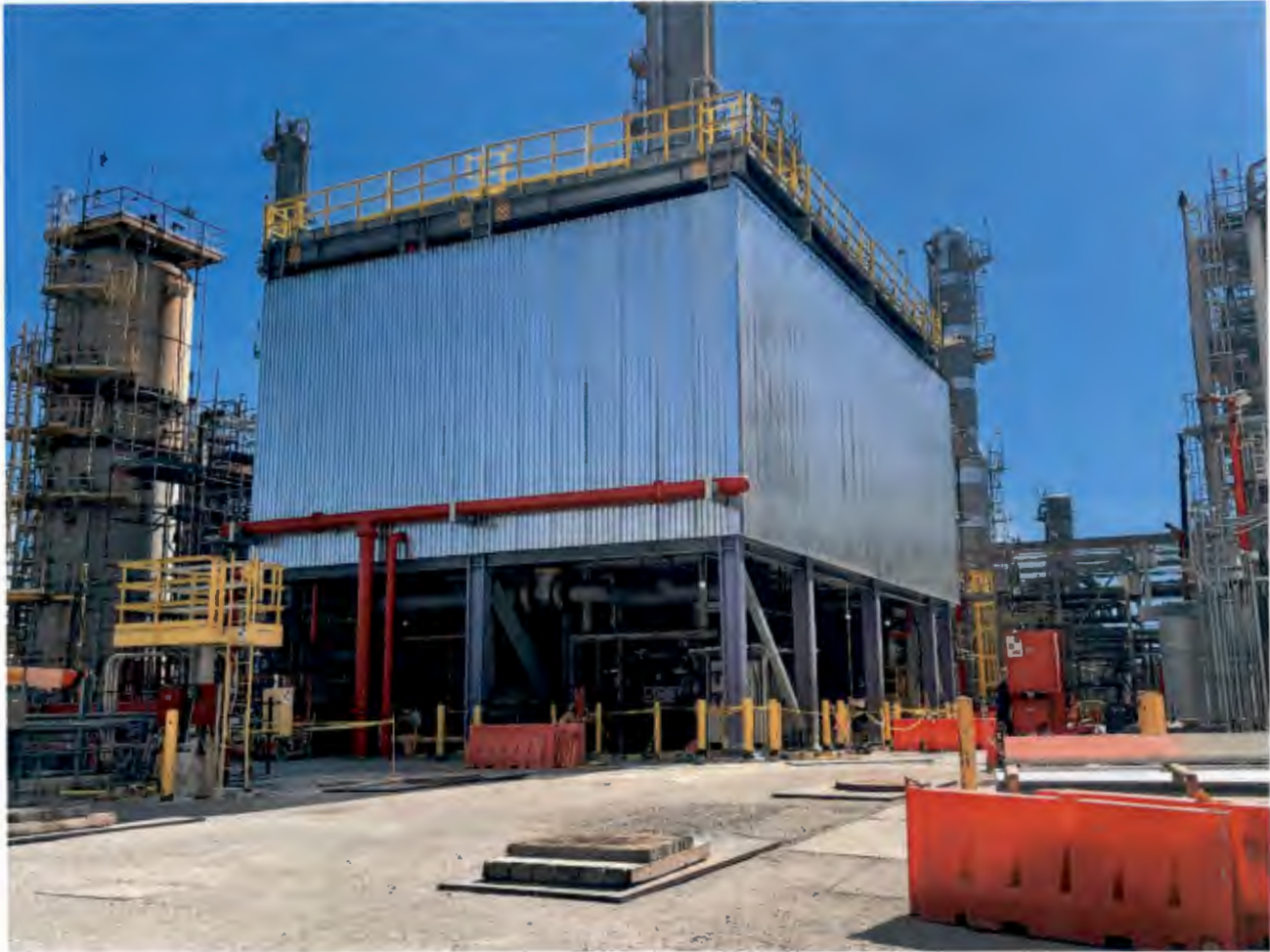
Structure North Wall View With Roof, North, and West Panels Installed
