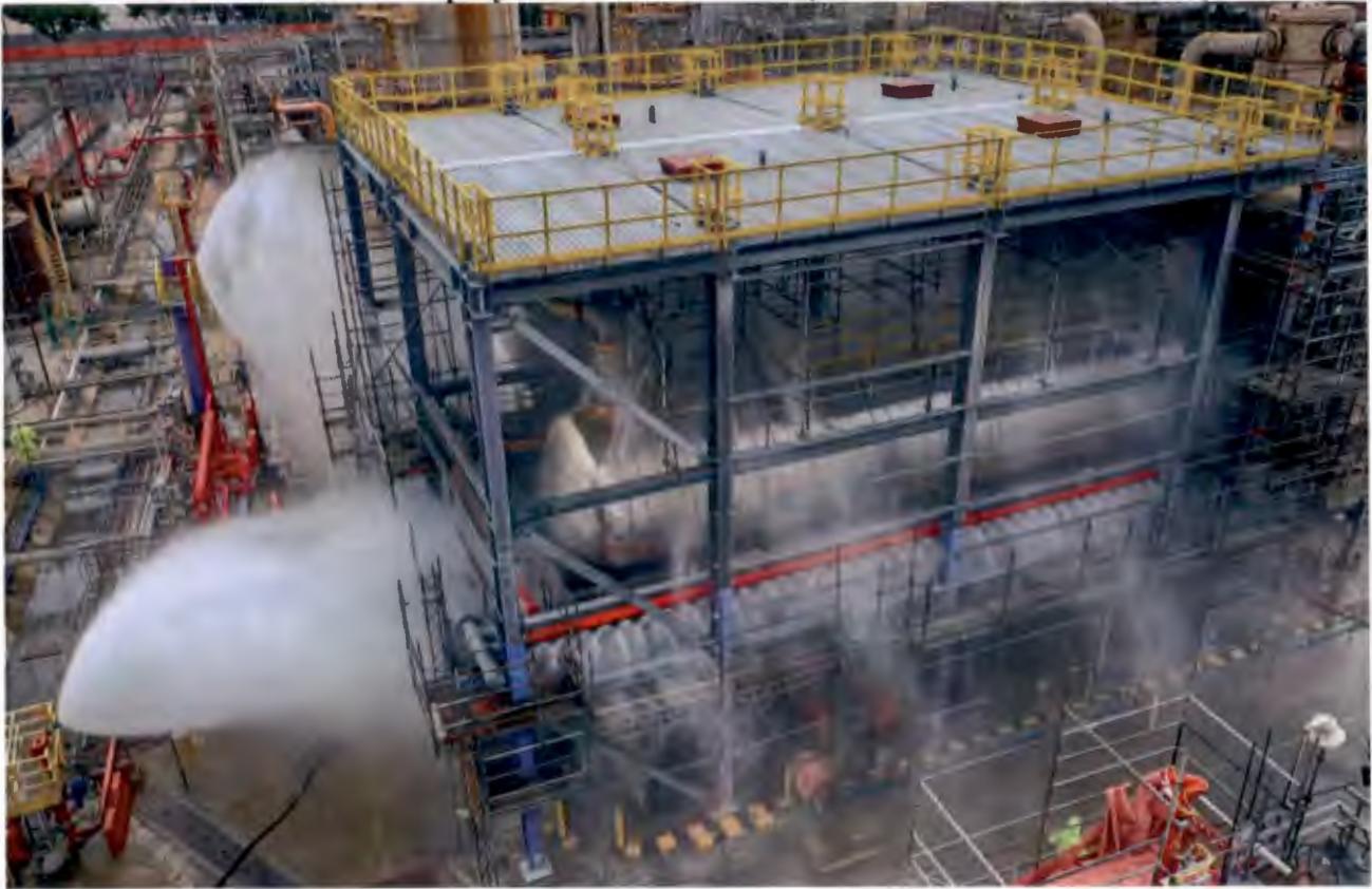
Dome Monitor and Spray Curtain – Flow Test (Before Side Panels Installed)
